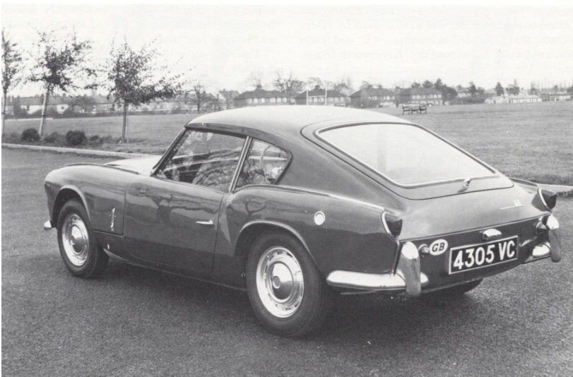
A shot of the "Spitfire Gt" taken in Coventry at her arrival from Turin: the roof shape and the rear door will remain identical in the final GT6, while a different design was adopted for the drip, the door windows (in this shot still without quarterlights) and for the position of the fuel cap.
